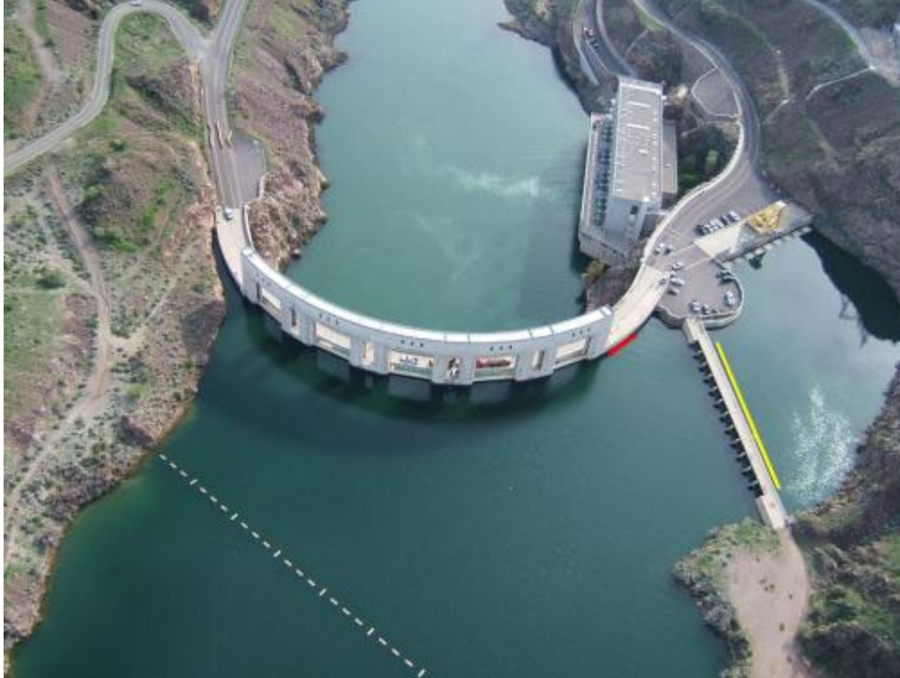
Figure 1: Ariel view of Parker Dam. Yellow line is the flowing water test location downstream of the trashracks. Red line is location of quasi-static water flow testing on the side of the dam.
