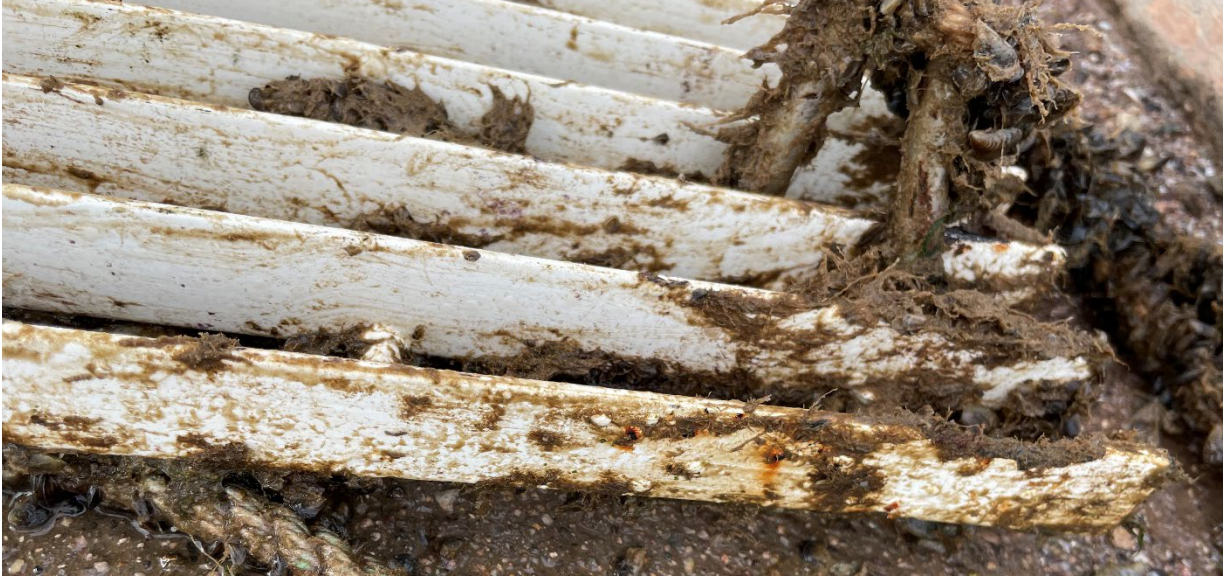
Figure 25: Corrosion present on edge of NuSil 9707 test grate, likely from damage.
