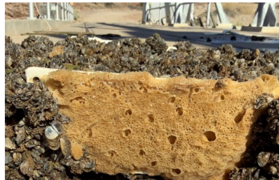
Figure 57: NDSU 8 in flowing conditions during January 2022 covered in sponge organism.
