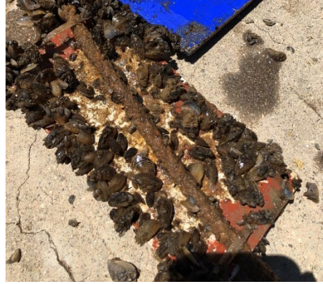
Figure 66: NDSU 9 quasi-static plate with damaged backside allowing for mussel fouling.
