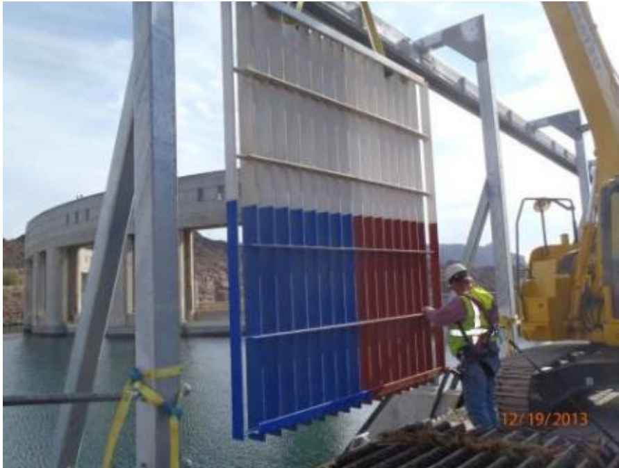
Figure 102: Trashrack during installation in 2013.
