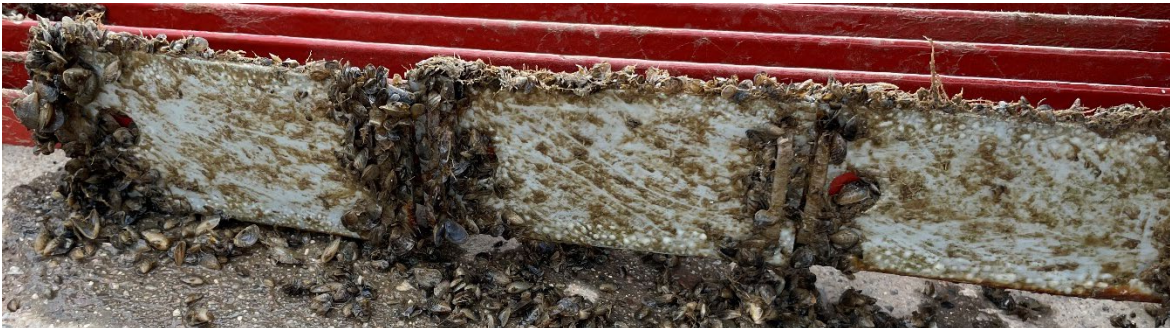
Figure 80: Formulation F panels after cleaning during July 2022 inspection.
