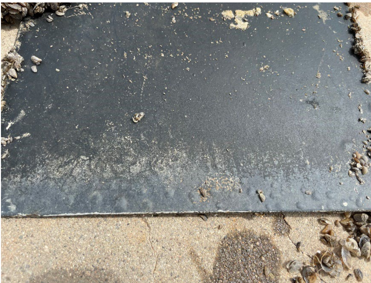
Figure 48: Blister on bottom of BioClean static plate which were observed during July 2022 inspection.
