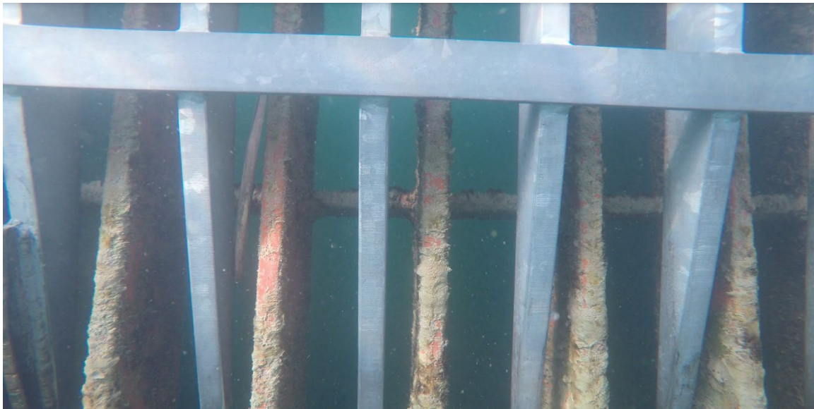
Figure 104: Sigmaglide 890 on trashrack. Coating is in good condition.
