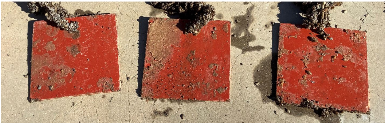
Figure 50: Hempel X3 Quasi-static test plates with fouling around damaged edges and fouled with sponge organism during January 2022 inspection.
