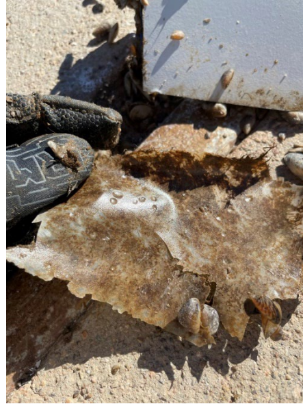
Figure 62: Delaminated topcoat from NDSU 3. Blisters can be seen in the film.
