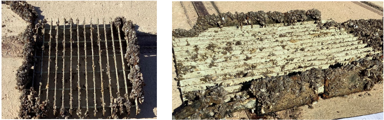
Figure 16: Top and side view of Silicone Solutions F-23 during January 2022 inspection.
