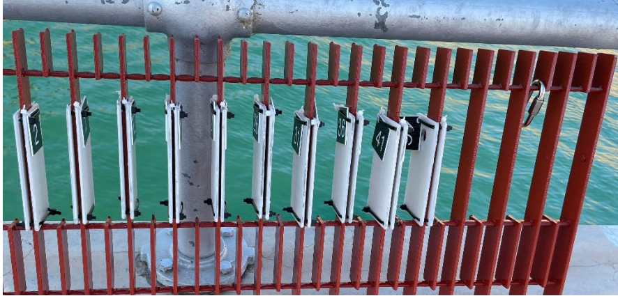
Figure 88: PNNL panels prior to install for testing during January 2022 inspection.
