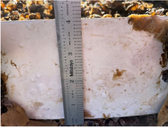
Figure 58: Blisters on NDSU 8 flowing water panel during January 2022 inspection.
