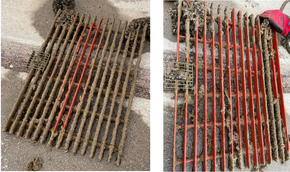
Figure 51: Hempel X3 dynamic test grate, covered in colonial hydroid, before and after cleaning during July 2022 inspection.
