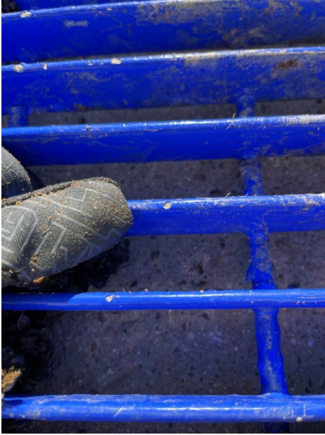
Figure 38: Damage to flowing water InterSleek 970 test grate in the form of small chips.
